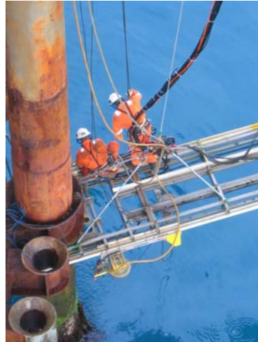
Cutting / removal of structures
