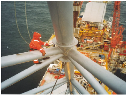
Up in the flare stack
