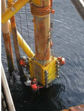
Installation of steel structure
