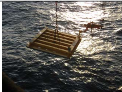
Installation of wave protection
