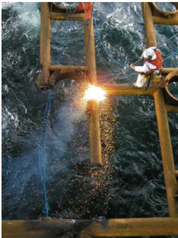
Removal of conductor frame
