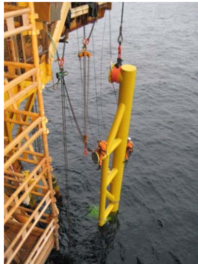
Mounting of riser protection
