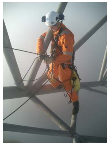
Wind braces in the flarestack
