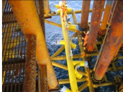
Installation of conductor frame
