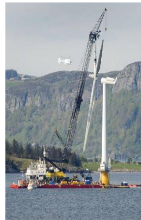
The Hywind experience Inshore assembly = Low cost & risk
