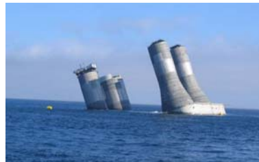
Concrete GBS – Sakhalin 2
